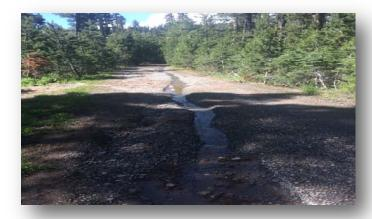
Corrective actions on Bucks Pasture Trail (17E17) have been identified. Trail maintenance on approximately 250 ft. of trail will re-establish drainage features and be done by a trail crew with hand tools. The work to scheduled to occur in September, 2017.
